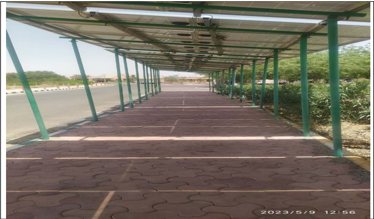
Solar panel in the campus on footpaths helps in electricity generation as well as provide shadow to users
